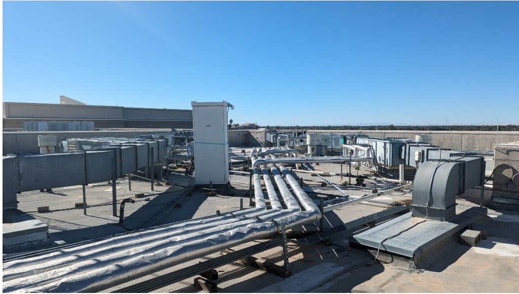
3. Overview of Building G roof.
