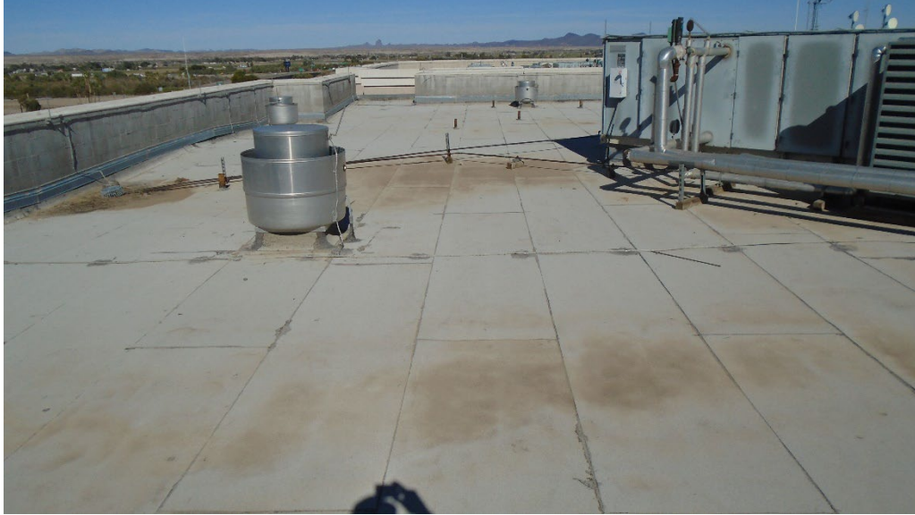
1. Overview of a Building F roof.
