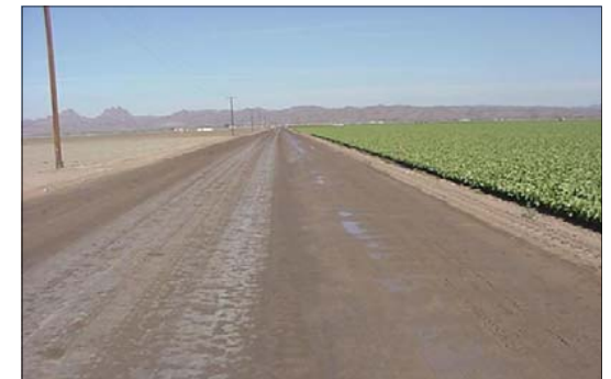
County roads are routinely maintained by Yuma County Public Works. Over watering can cause damage to roads and accidents.
